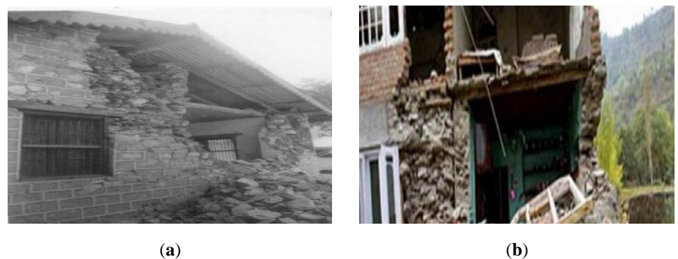
Figure 2. Junction failure during Kashmir Earthquake [9].
